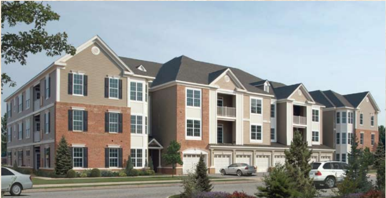
The Lennar Centre Place at Edison is a redevelopment of a former military arsenal in Edison, New Jersey.
